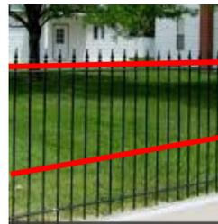
This fence could be retrofit by removing the finials (pointed tops) and adding a cross member at the top and the two foot mark.
