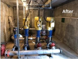
The switch to VFD control allowed for reduced power consumption and more consistent control of the water pressure. The current connections consume the full allotment of licensed water from the well and so no further connections can be considered at this time.
