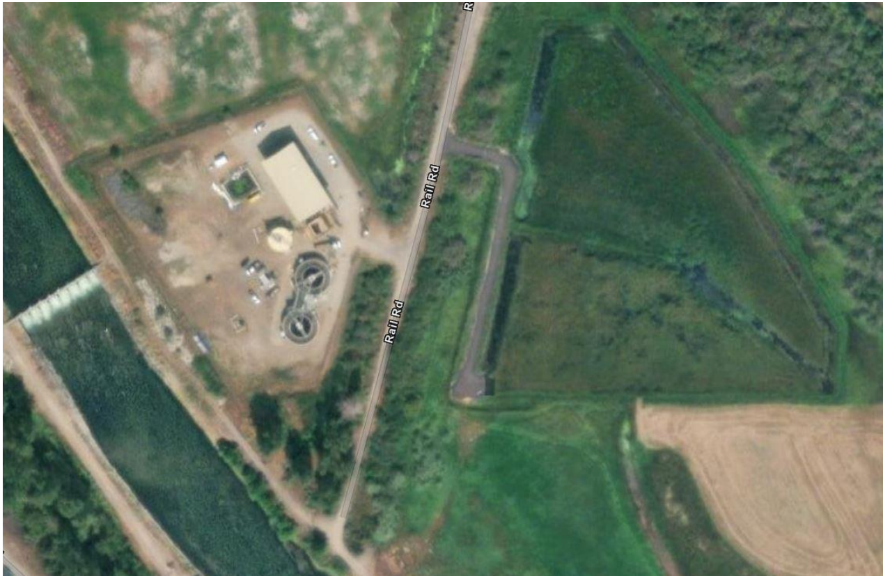
Aerial view of Okanagan Falls Biological Nutrient Removal Wastewater Treatment Facility showing centrifuge dewatering facility under construction in 2021 and polishing wetland located on the right side of Rail Rd.
