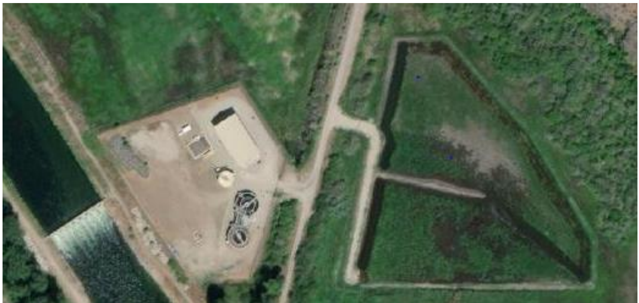
Aerial of Okanagan Falls wastewater treatment facility and constructed polishing wetland.
