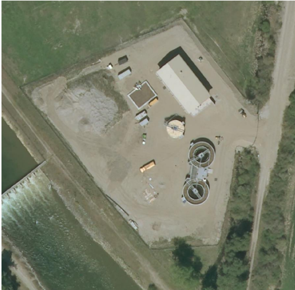
Aerial view of Okanagan Falls biological nutrient removal wastewater treatment facility
