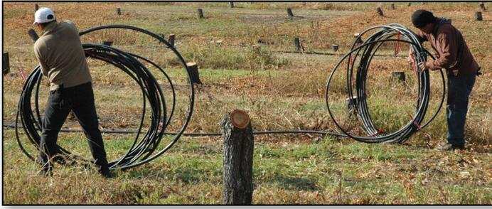
All surface materials (wire, irrigation, treated posts) must be removed prior to excavation/pulling of trees
