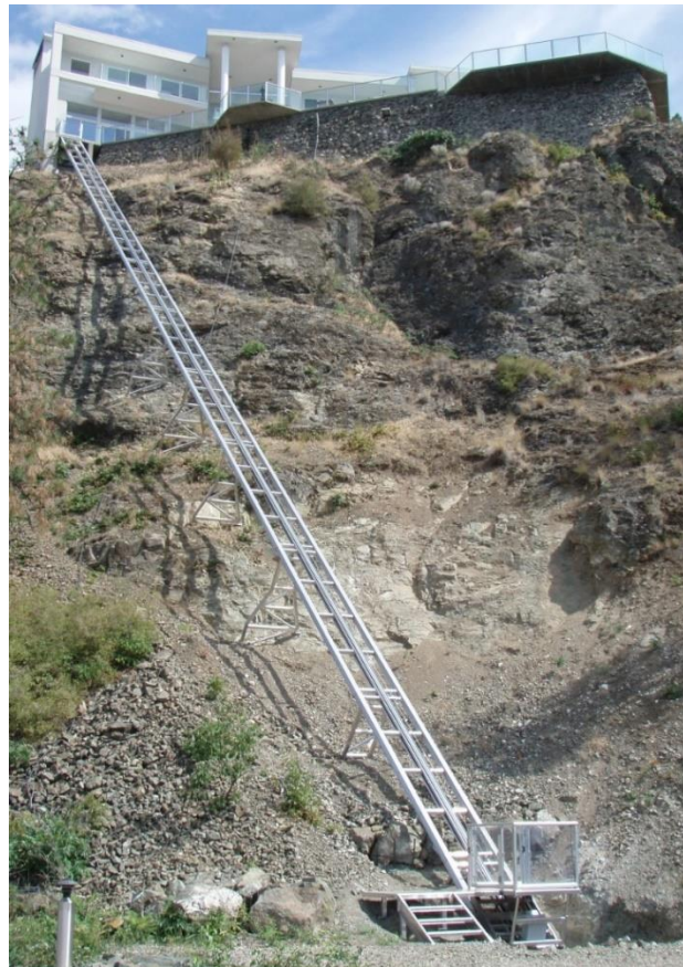
Photo 8. View of example tram to illustrate how it hovers over the landscape and the minimal permanent footprint associated with the helical screws.
