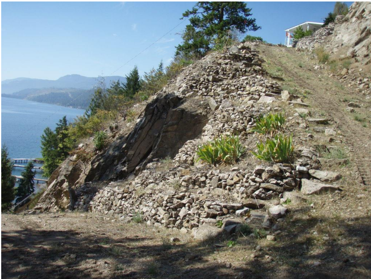
Photo 10. View of example trail/road to illustrate how extensive cuts and fills and switchback can severely alter the landscape in order to achieve the required grades.
