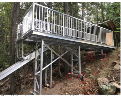
Photo 11. View of a tower bracket on two piles and their minimal permanent footprint.
