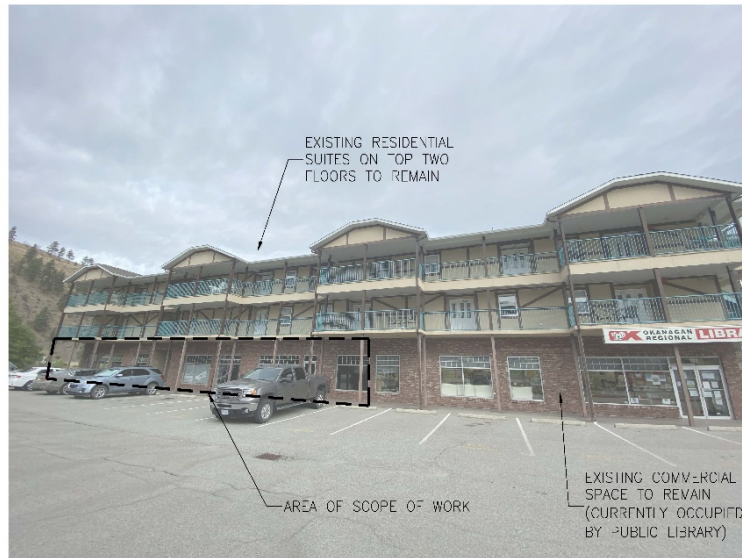
EXISTING BUILDING (SOUTH EXPOSURE) ELEVATION PHOTO NOT TO SCALE
