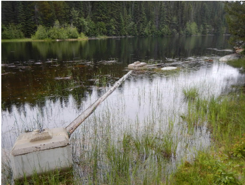
Photo A14: Elinor Lake South Dam, Log Boom
