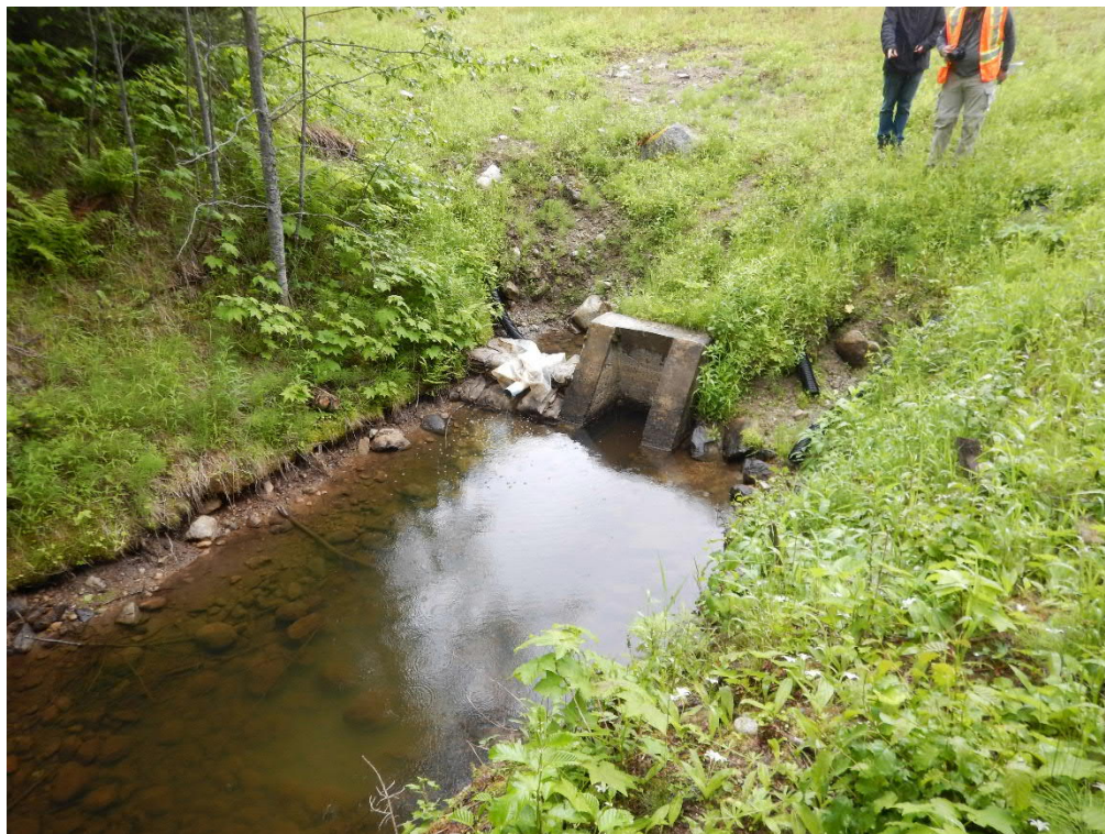
Photo A6: Elinor Lake South Dam Outlet Works, Tailrace Channel, Seepage on Right of Structure
