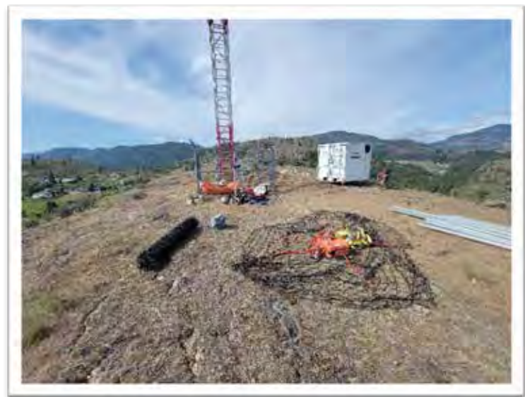
Figure 1: Kaleden Repeater Tower Construction site
