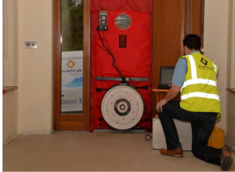
Air-Tightness Testing • Achieve minimum performance levels
