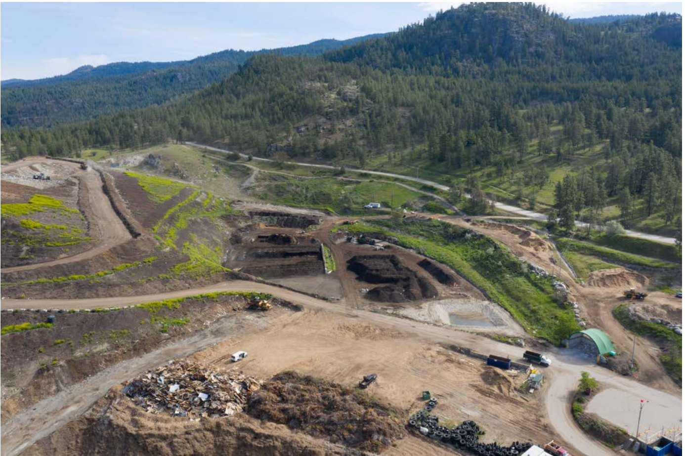
Wastewater Solids Composting Operation
