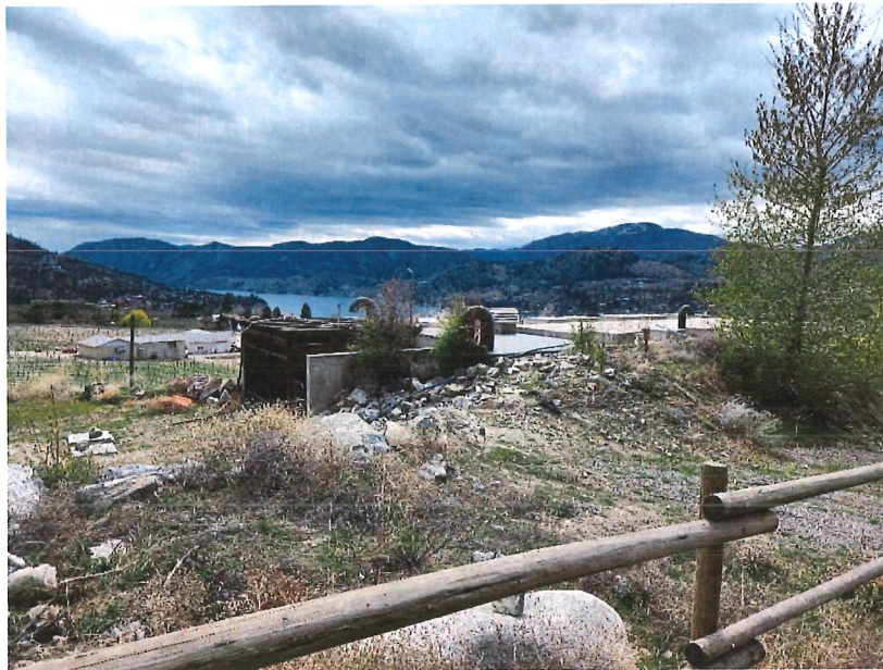
Figure 9: Vintage Views WWTP: Existing fencing in the foreground
