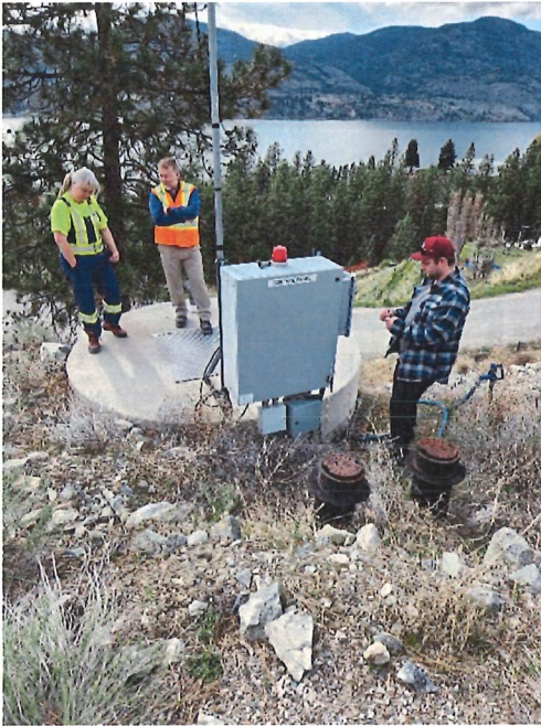
Figure 14: Existing lift station
