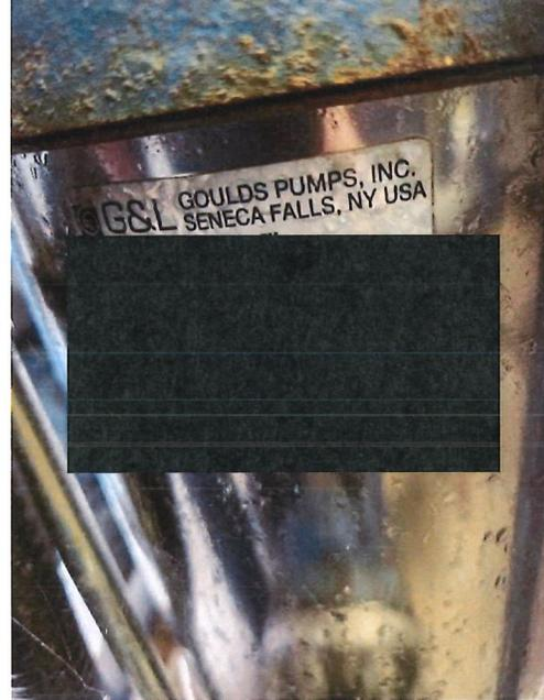
Figure 24: Christie Mountain Pumphouse: Corrosion visible on pump electrical motor frame
