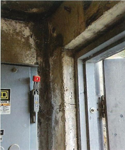
Figure 19: Christie Mountain Pumphouse: Cracks in concrete walls
