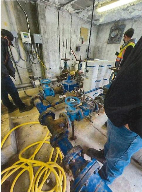
Figure 15: Sunnybrook Pumpstation: Corroded pipework and valves, untidy tubes, dirty ceiling
