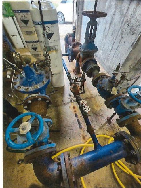
Figure 16: Sunnybrook Pumpstation: Corroded steel pipework and corroded valves
