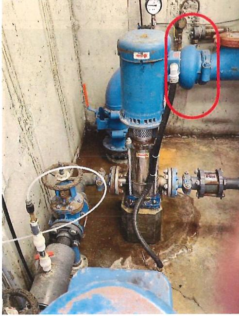
Figure 23: Christie Mountain Pumphouse: Pressure Reducing Valve requiring testing and refurbishment.
