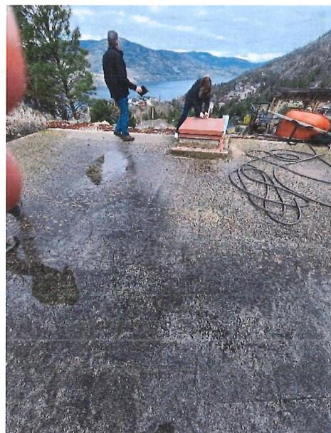
Figure 33: The roof slab of the Apple Court Reservoir is covered with lichen and moss, but generally in good condition.
