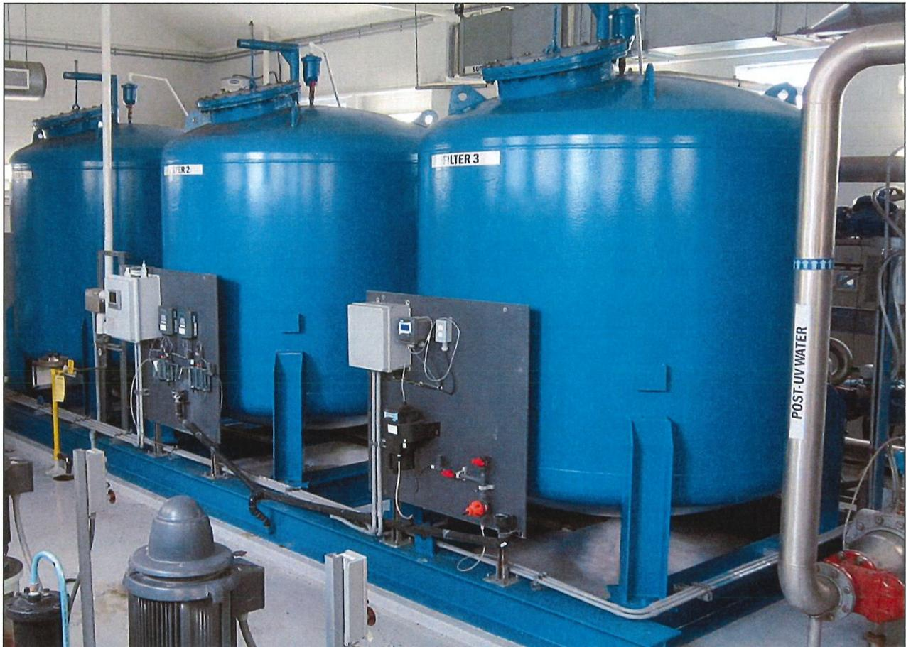
Figure 34: A typical pressure filter installation
