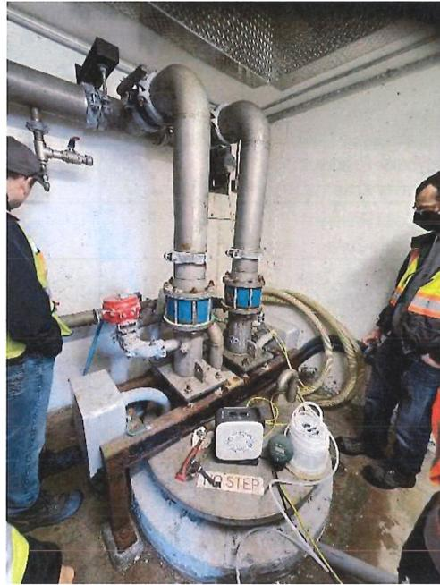
Figure 8: Lakeshore Pumphouse: Wet well and pump headers
