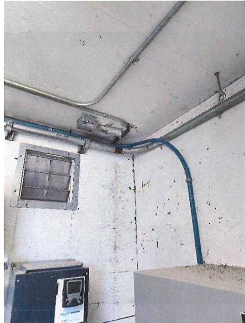
Figure 14: Lakeshore Pumphouse: Bottom Level: Leak through roof
