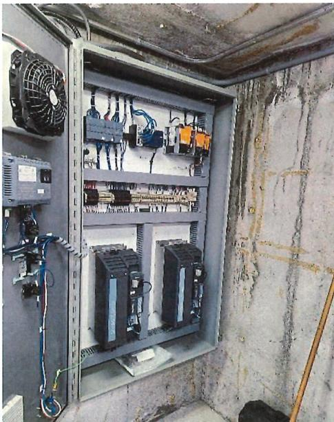
Figure 17: Sunnybrook Pumpstation: 600 Volt Variable frequency drives (VFDs) and programmable logic controller (PLC) in the same box
