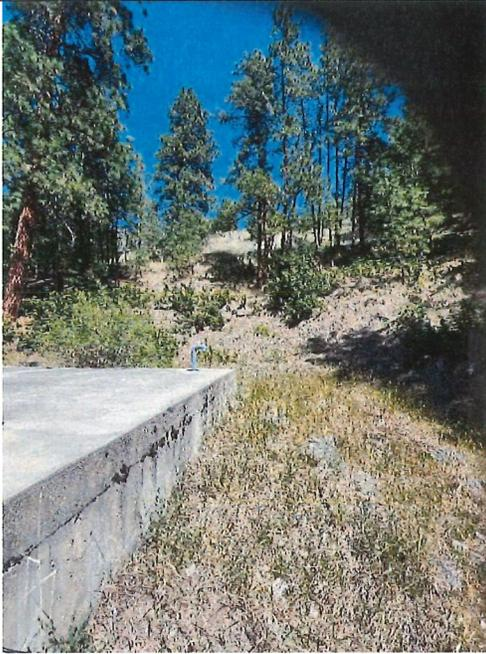
Figure 29: Sunnybrook Reservoir: Top of the concrete walls and roof slab on the left; stormwater channel on the right
