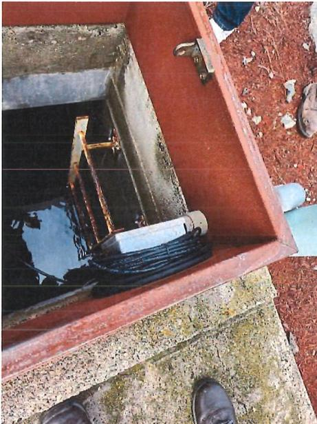
Figure 32: Apple Court Reservoir: Internal ladder shows signs of corrosion.
