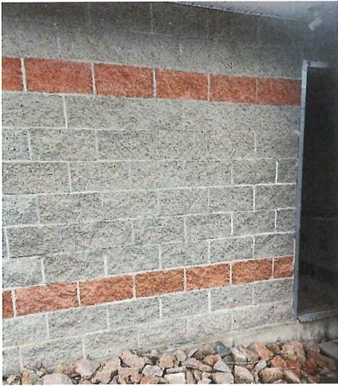
Figure 25: Apple Court Pumphouse: Cinder block walls are generally in a good condition.
