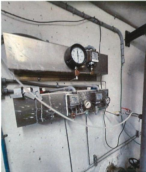
Figure 11: Lakeshore Pumpouse: Bottom Level: Mechanical pressure gauges and tubes
