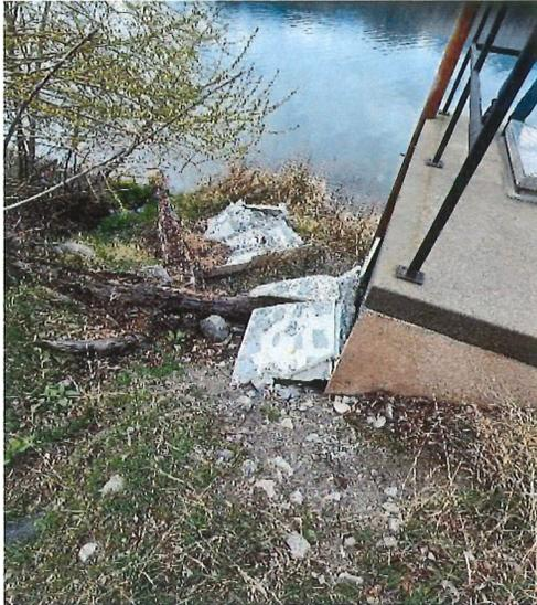
Figure 9: Lakeshore Pumpouse: Disintegrating outer walls.
