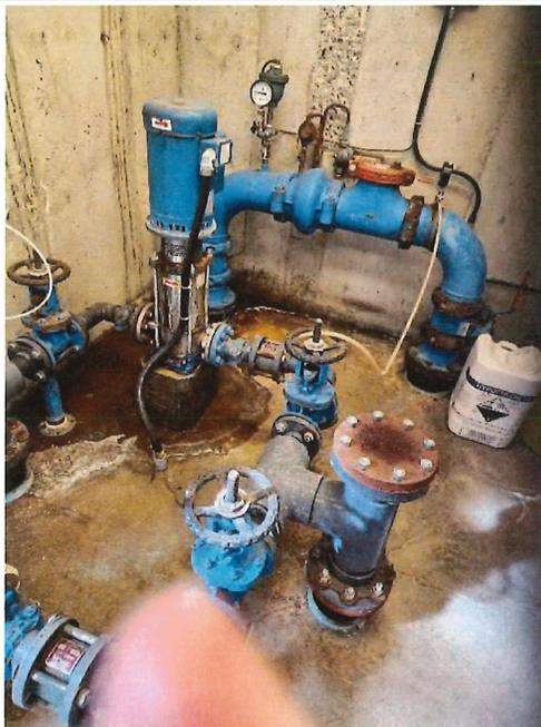
Figure 21: Christie Mountain Pumphouse: Water leaking from pump
