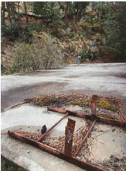
Figure 31: Sunnybrook Reservoir: Corroded steel ladder
