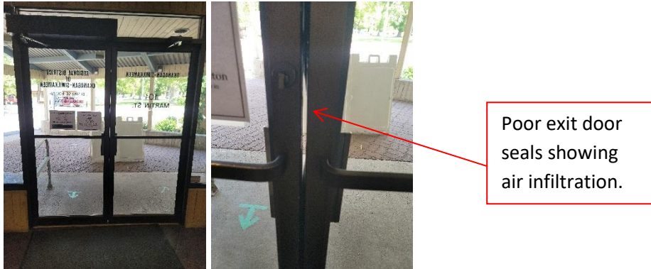
Figure 10: Existing Door Seals
