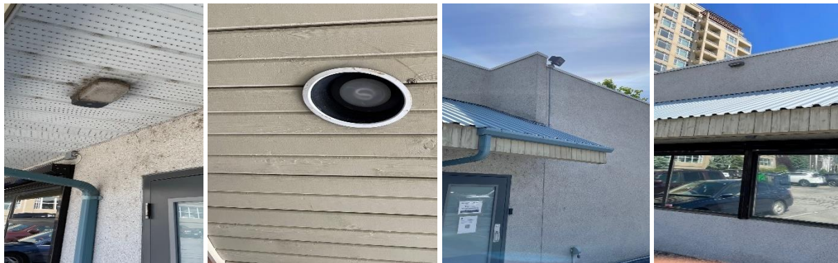
Figure 13: RDOS Office External Lighting
