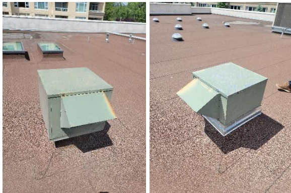
Figure 8: Existing Two (2) DELHI Exhaust Fans on Roof
