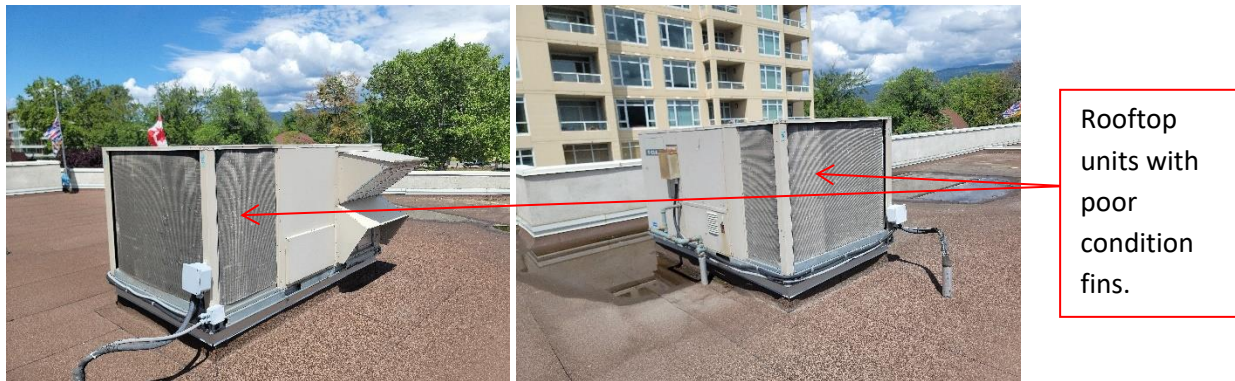
Figure 6: Typical Existing LENNOX Gas Fired Rooftop Units
