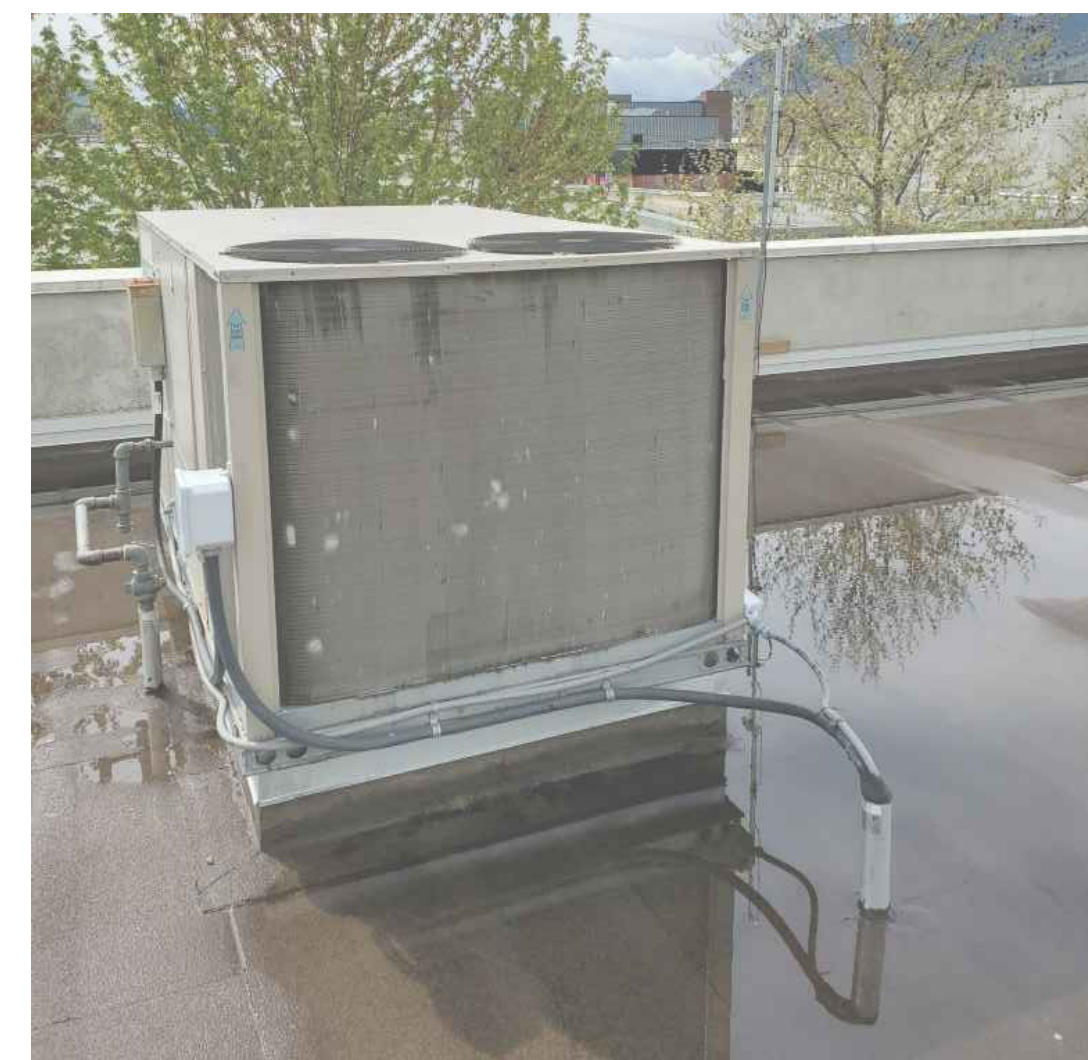
2 EXISTING ROOFTOP UNIT DETAIL 1 (TYP.) M-3 SCALE: NTS
