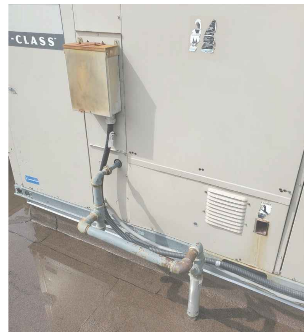
3 EXISTING ROOFTOP UNIT DETAIL 2 (TYP.) M-3 SCALE: NTS
