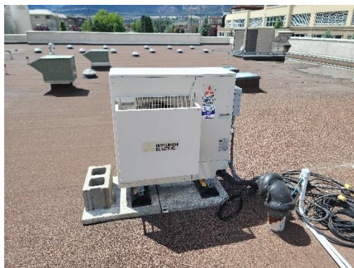
Figure 7: Existing MITSUBISHI Split System – Condensing Unit on Roof
