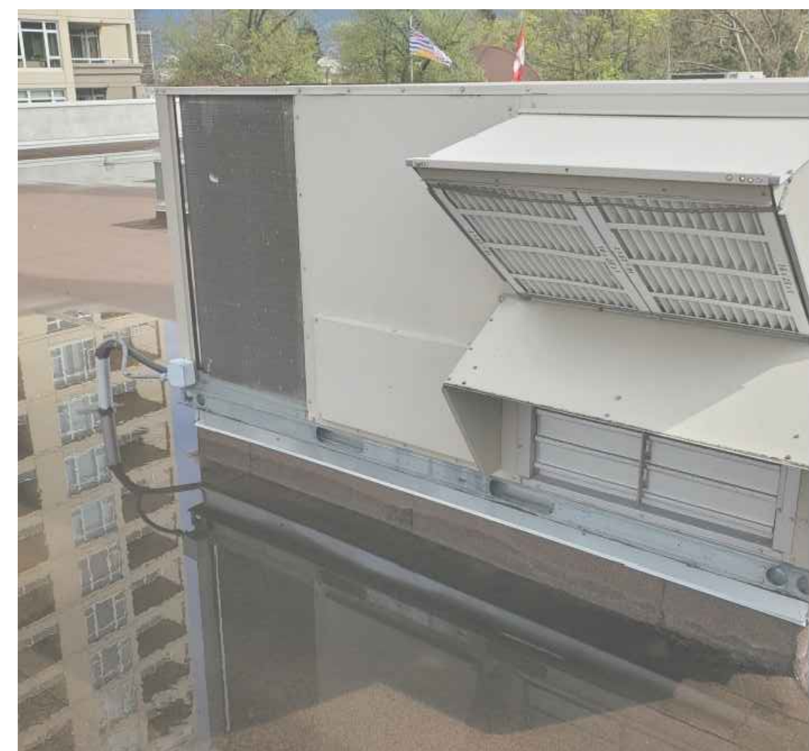
4 EXISTING ROOFTOP UNIT DETAIL 3 (TYP.) M-3 SCALE: NTS
