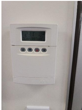
Figure 11: Typical Existing Wall Mounted Thermostat
