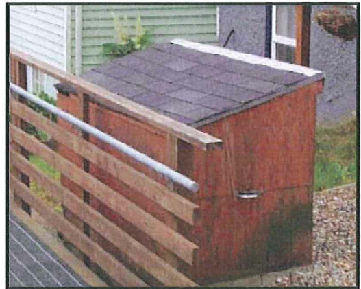
Wooden enclosure. Strengths: Seamless construction, metal flashing on seams, and minimal overhang of roof.
