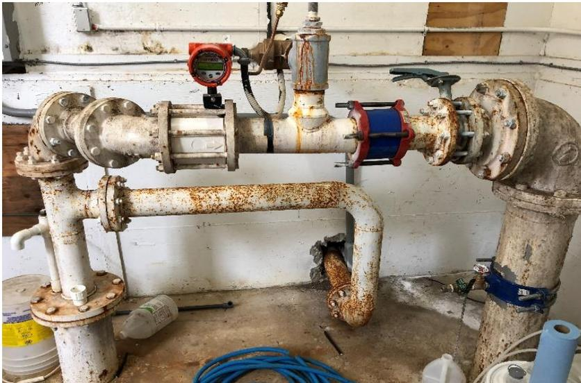
Figure 2 Inside Willowbrook Pump Station (Bottom Left: original well head; Bottom Centre: 2006 Well supply; Top Centre: Inline flowmeter air release valve, and isolation valve; Bottom Right: Common discharge leaving Pump Station)
