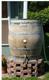
A nicely installed rain barrel. **But**, in the Okanagan, it is not recommended to use a wooden barrel. The intense summer heat dries the wood and they leak.
