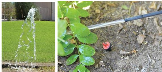
*broken sprinkler head & missing drip emitter*
