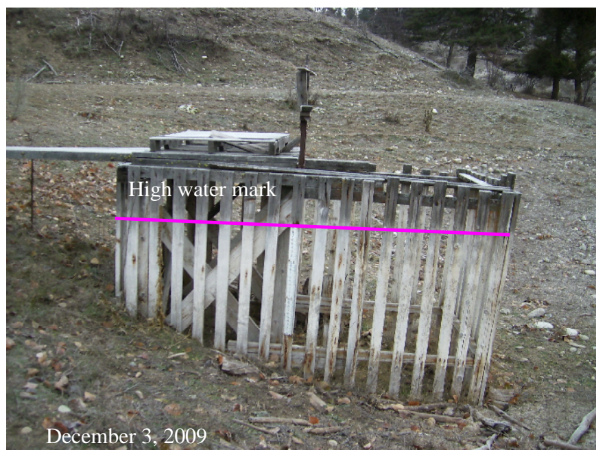
Photo D1. Protective wooden structure around sluice gate inlet.
