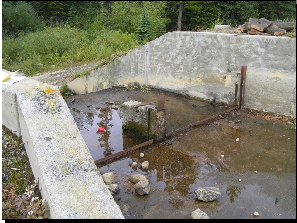
Photo 1 Big Meadow Lake Dam — Spillway structure with Stop logs removed
