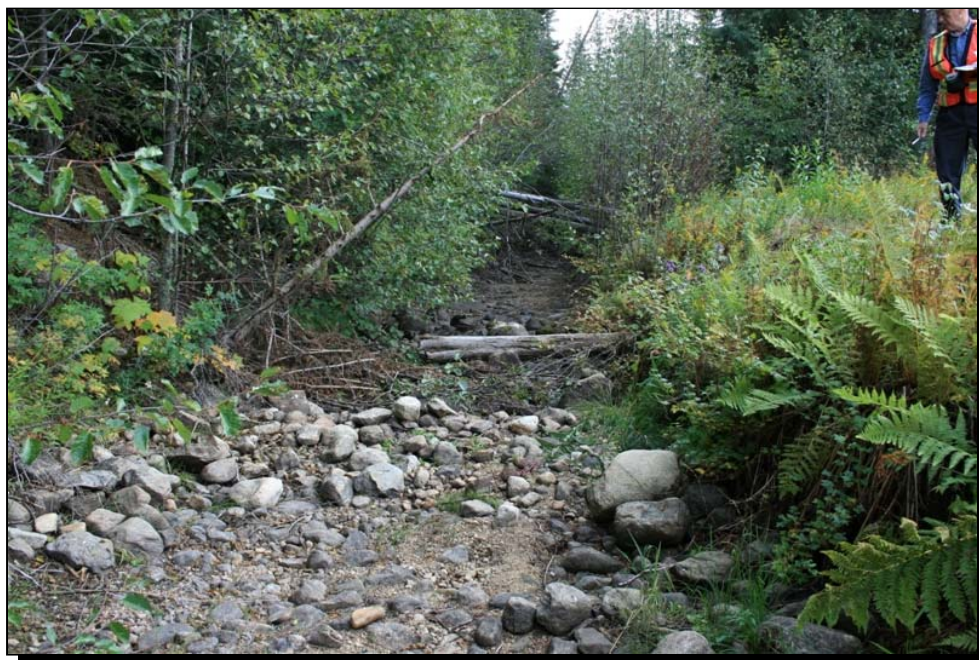
Photo 6 Elinor Lake South Dam — Wood debris in spillway channel
