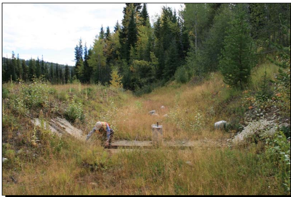
Photo 8 Naramata Lake Dam — Spillway Weir, stop logs removed
