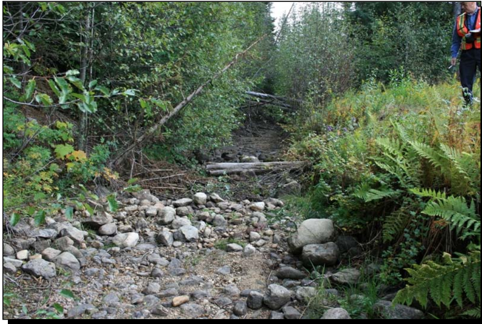
Photo 13 Elinor Lake South Dam — Wood debris in spillway channel
