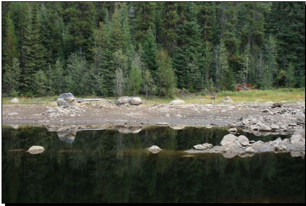
Photo 14 Elinor Lake South Dam — Spillway channel entrance, no log boom and accumulation of silt
