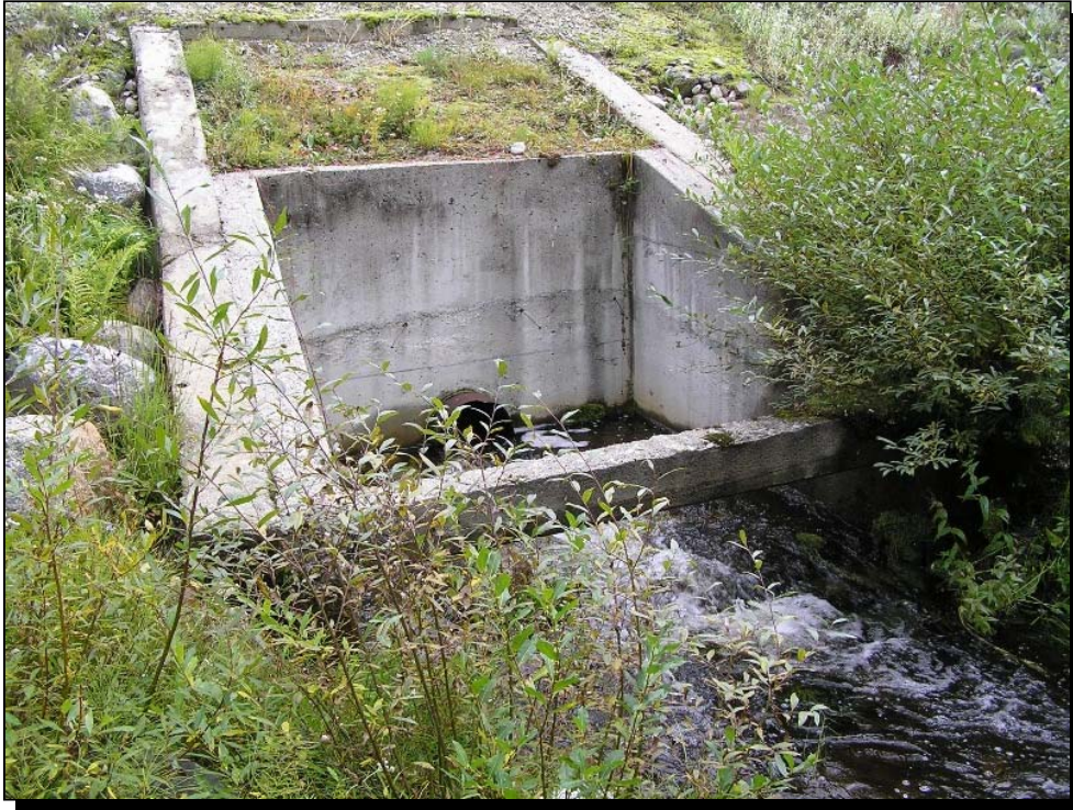
Photo 9 Big Meadow Lake Dam — Low-level outlet structure
