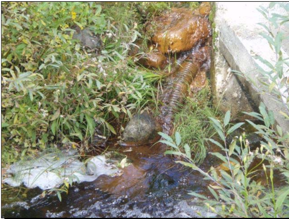
Photo 10 Big Meadow Lake Dam — Seepage from right of low-level outlet structure
