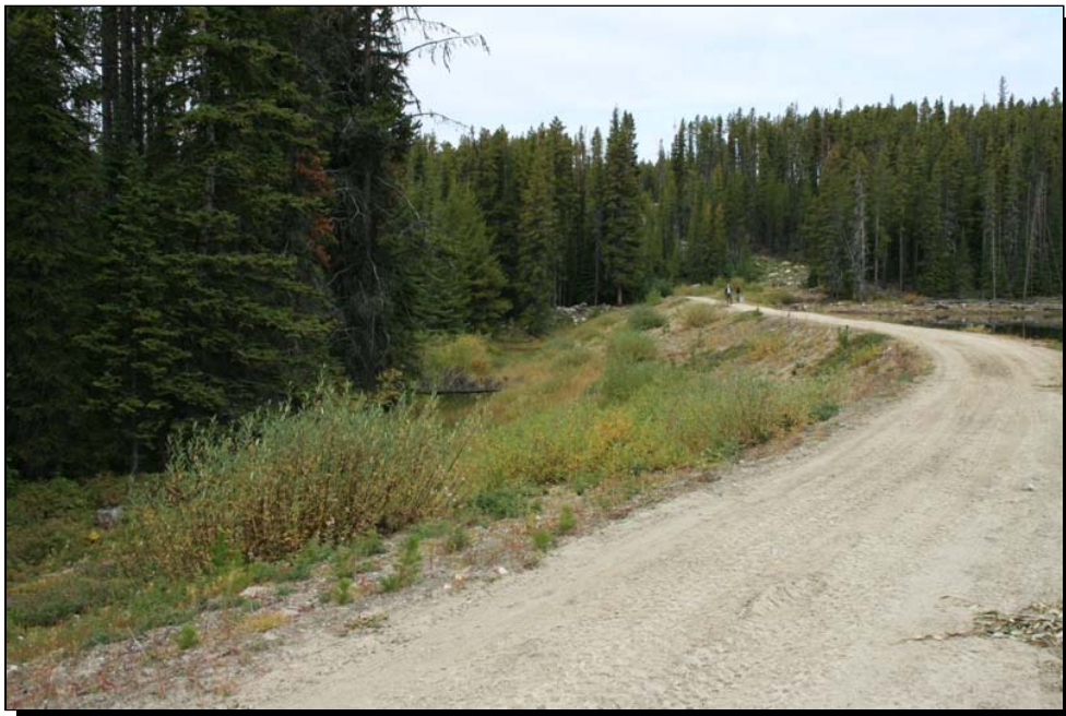
Photo 2 Big Meadow Lake Dam — Downstream Face from left abutment
