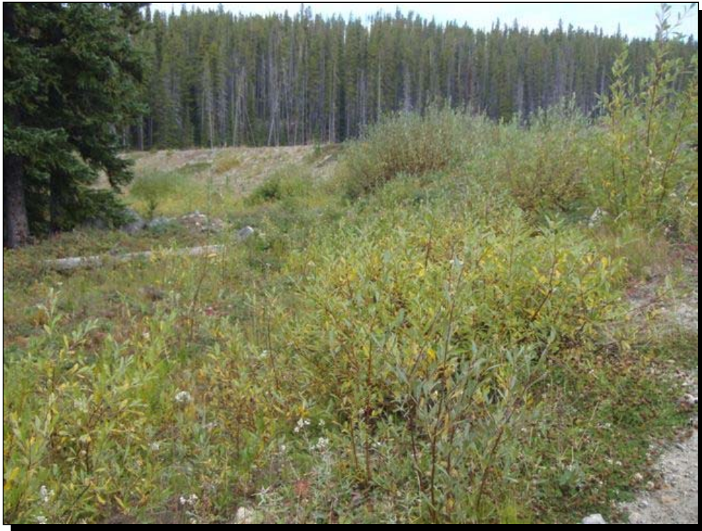
Photo 3 Big Meadow Lake Dam — Vegetation growing on left side of Downstream Face
