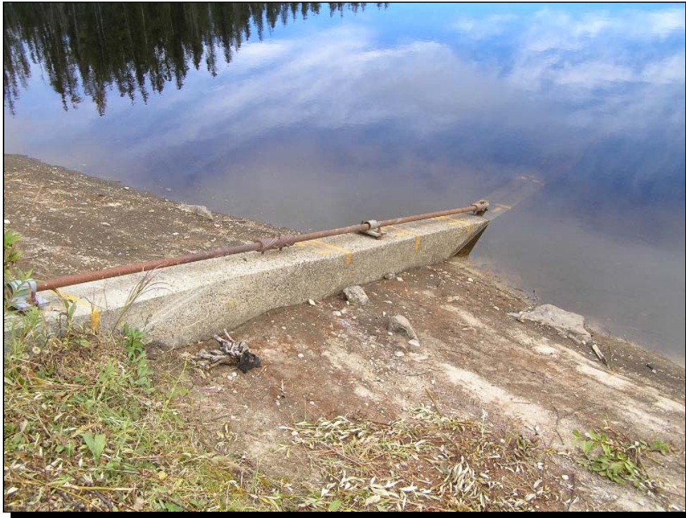
Photo 5 Big Meadow Lake Dam — Intake Structure Stem Guide
