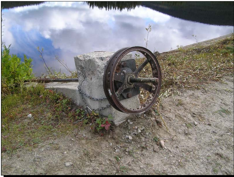
Photo 6 Big Meadow Lake Dam — Gate Hoist Head-block
