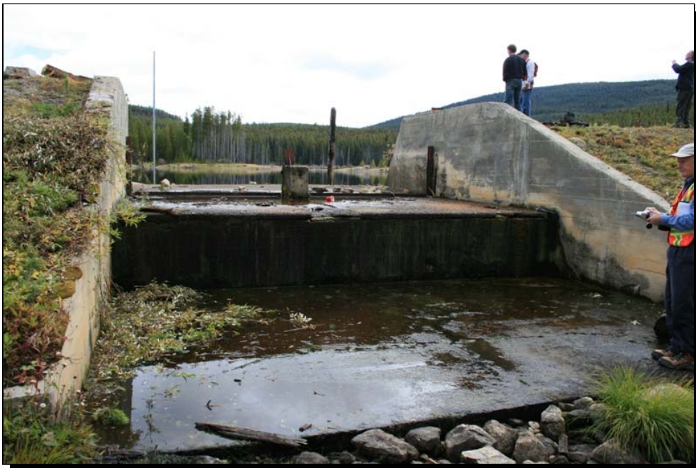
Photo 8 Big Meadow Lake Dam — Spillway structure downstream view
