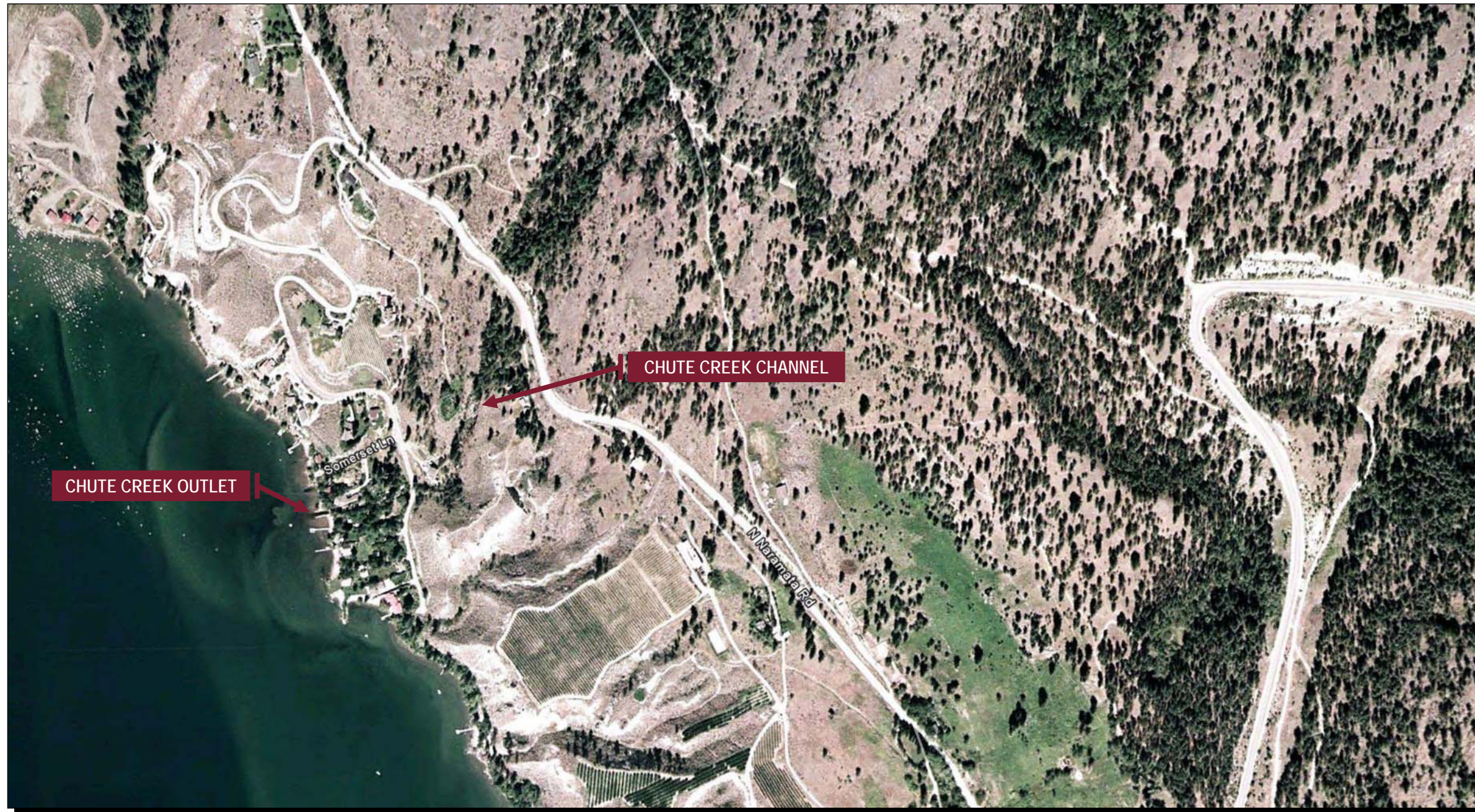
Photo 16 Chute Creek Outlet
