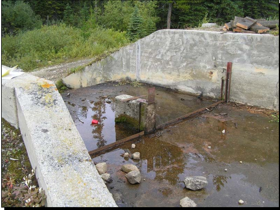
Photo 7 Big Meadow Lake Dam — Spillway structure with Stop logs removed
