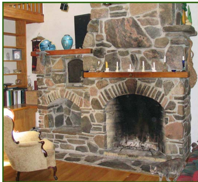
A beautiful and expensive fireplace, but notice the smoke stains on the stone arch and wooden mantel.
