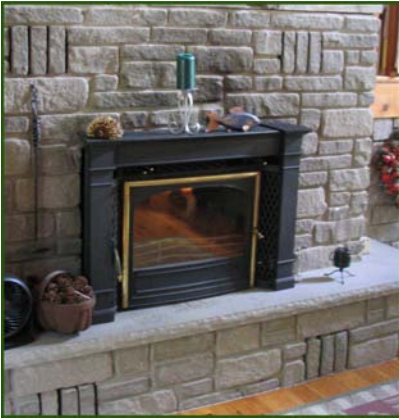
A fireplace insert converts a conventional fireplace into a heating system.
