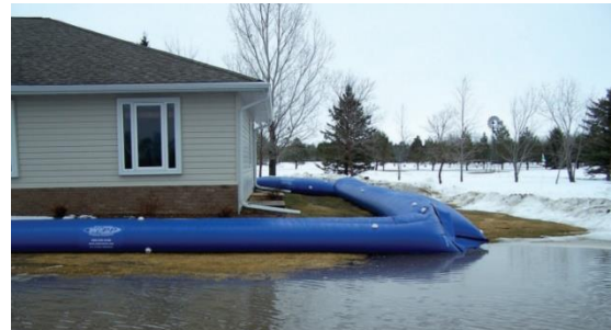
Figure 10.5 Example of a water-filled temporary barrier (FEMA, 2014)
