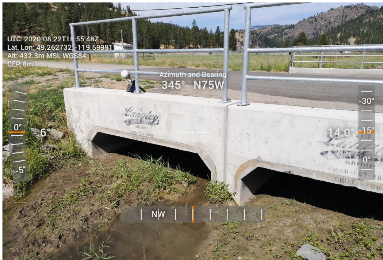
Photo 4 Box culvert along Carr Crescent in Willowbrook, showing sediment deposition at culvert
