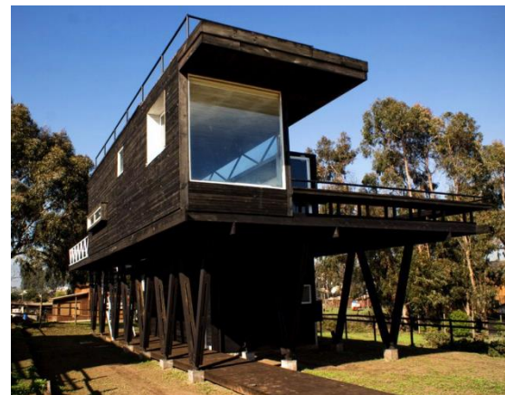
Figure 10.2 Example of elevated structure
