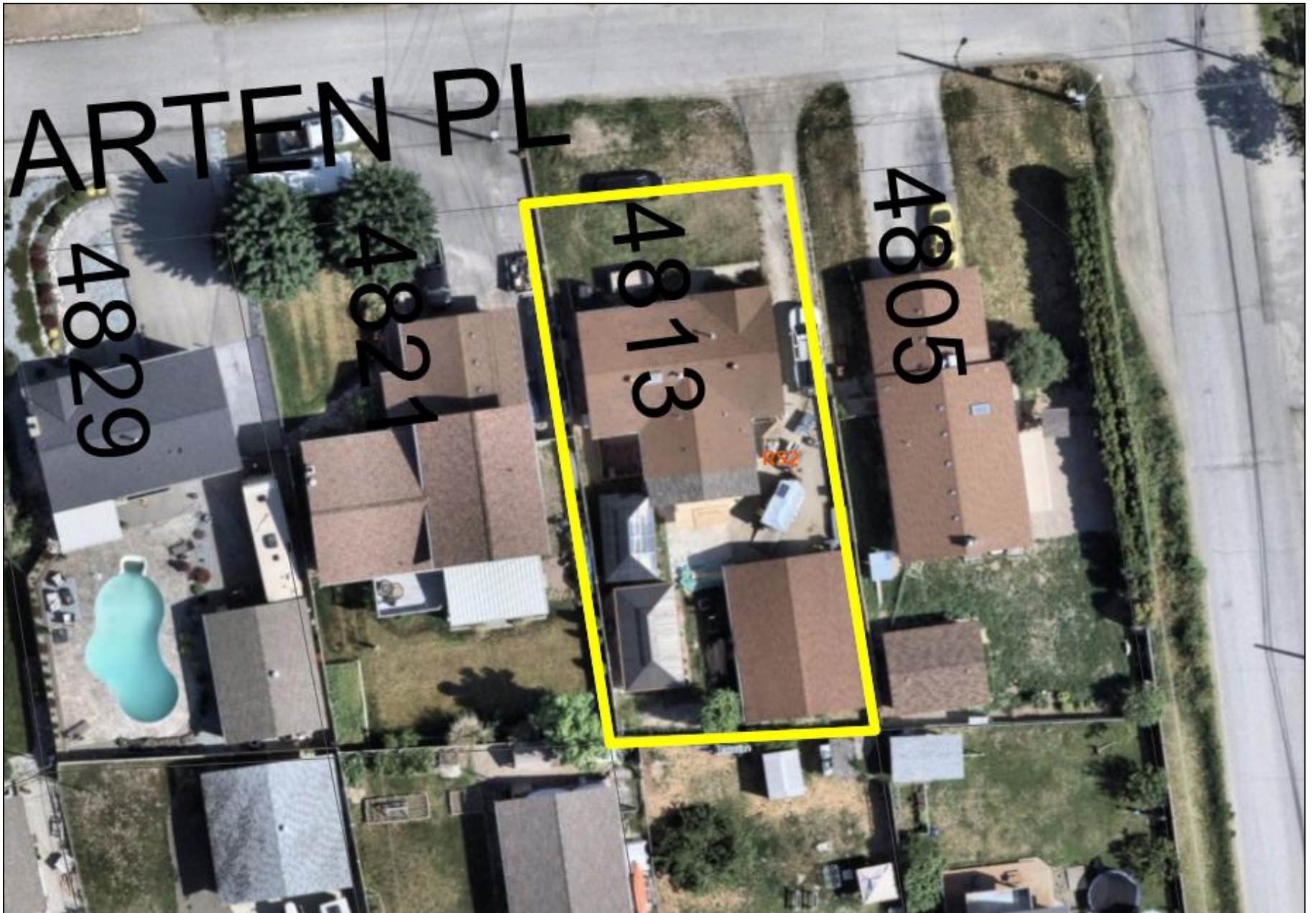
Attachment No. 1 – Aerial Photo
