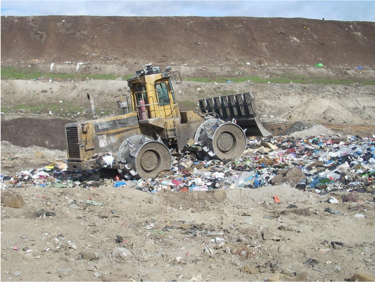
Compactor at Campbell Mountain Landfill (RDOS)
