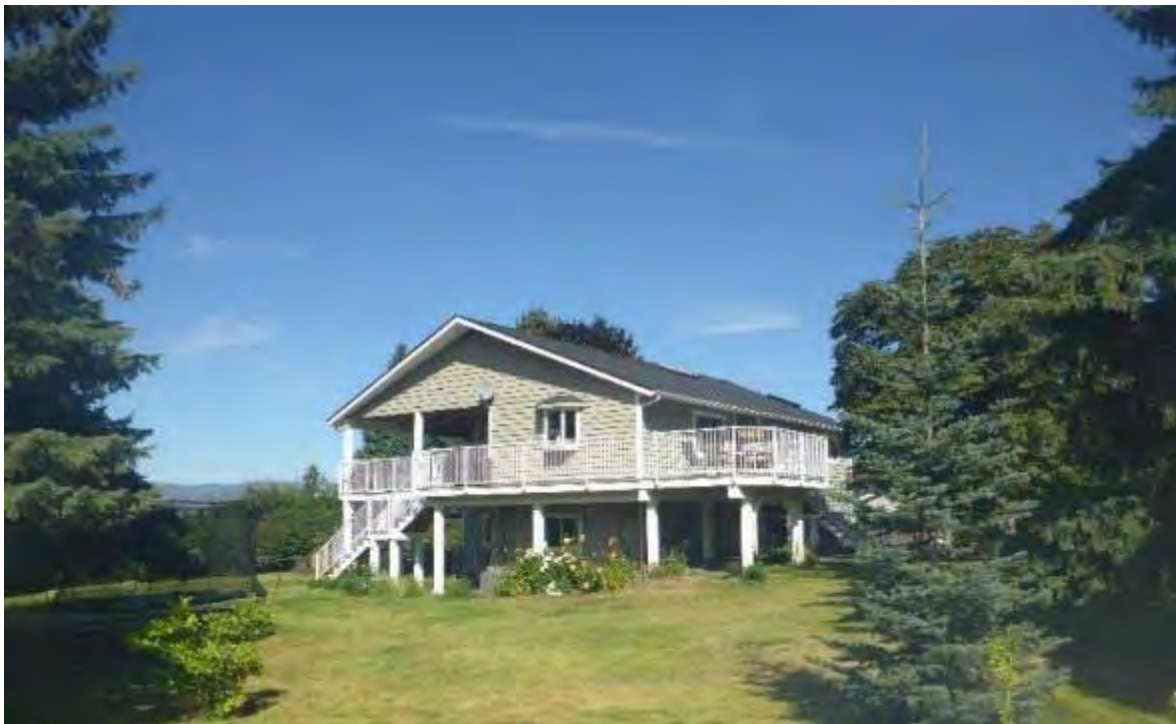
Figure 11: New homes are generally built to FireSmart building construction standards.
