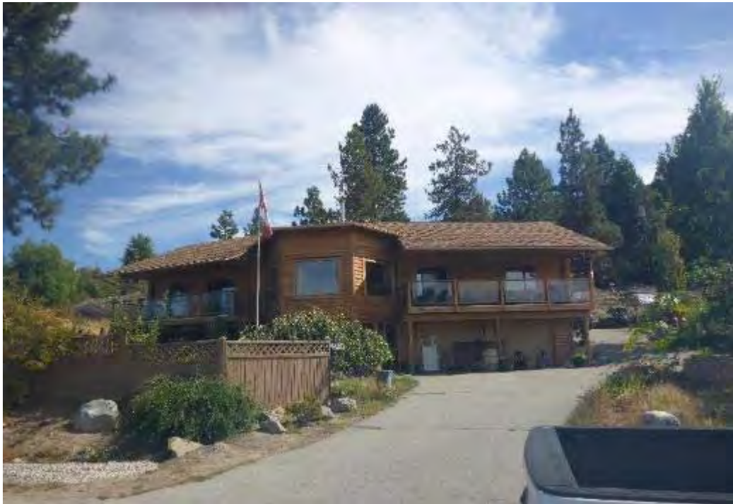
Figure 10. Non-compliant homes with cedar shakes and wood cladding
