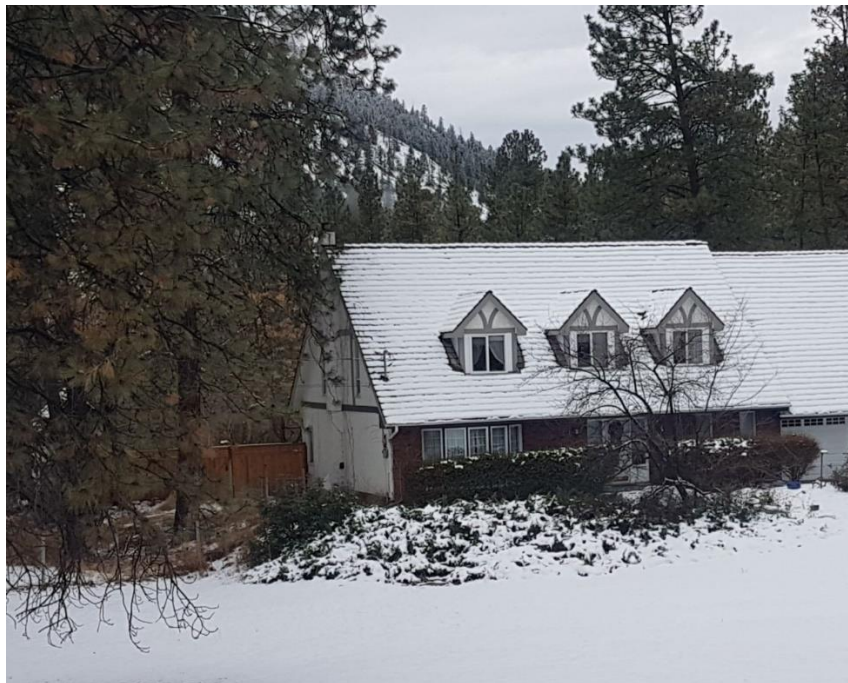
FIGURE 11 Several homes in Husula are characterized by the presence of volatile vegetation, such as cedar and juniper shrubs, in Zone 1. A wood fence abutting the home can provide a pathway for home ignition should the fence ignite. An unrated wood shake roof offers no fire-resistance.
