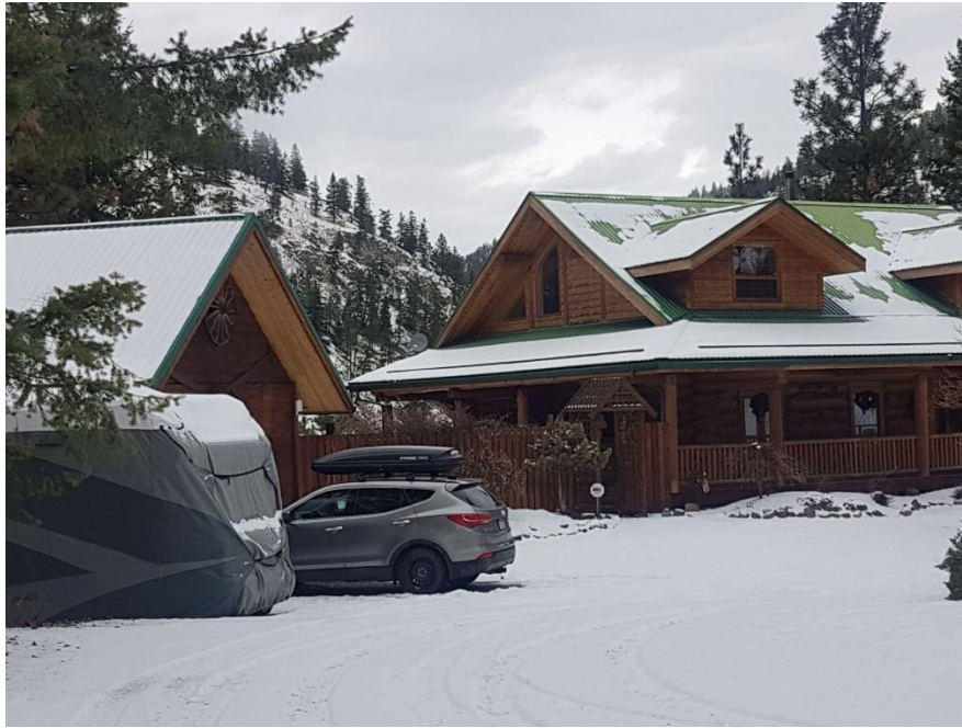
FIGURE 12 A rated roofing system, such as this metal roof, provides fire-resistance to embers. Any modern roofing system that has a fire-resistance rating can provide this protection. During a wildfire, particularly a high-intensity wind-driven fire, a tremendous amount of embers can be cast into the air, producing an ember shower or ember blizzard.
