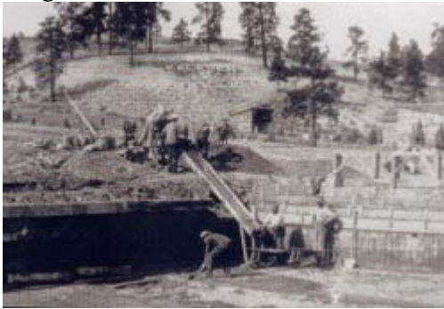
Early Stages of Construction
