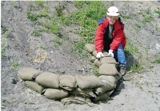
Corps employees demonstrate building a ring dike.
