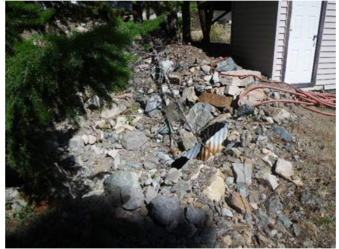
Photo B – Twin 1000mm bevelled culverts on dry Perley Creek passing under the driveway to the subject property. Wellhead shed to the right will be removed.
