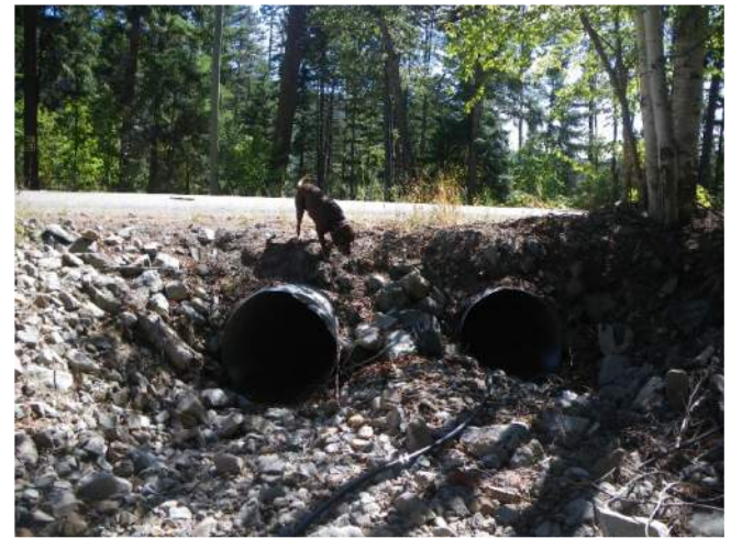
Photo D – Inlets of twin 950mm culverts under Coalmont Road. These culverts will have a lower capacity than the driveway culverts downstream (beveling increases capacity).
