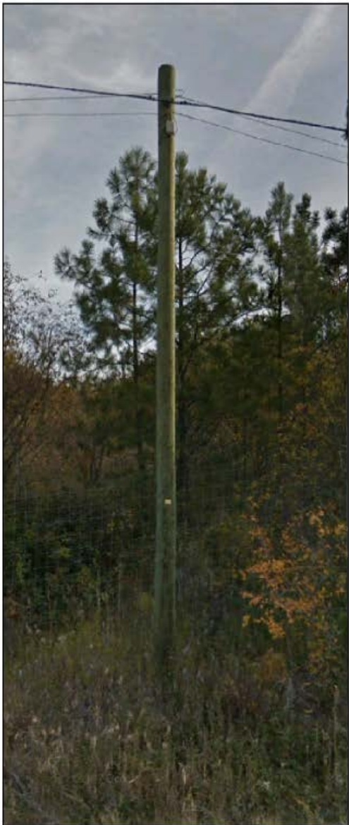
① EXISTING POLE PICTURE
