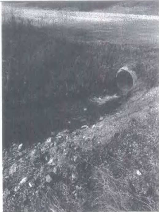
Photo 5 – 700mm culvert outlet on East side of Coalmont Rd
