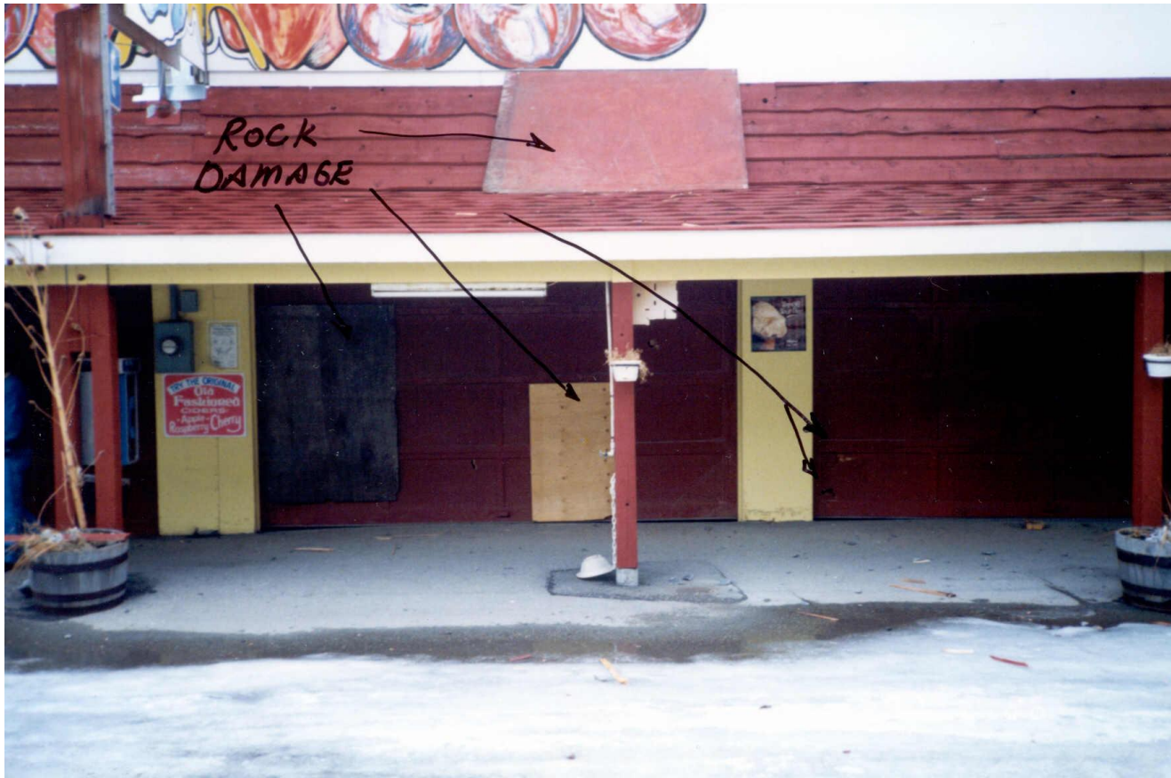
Photo 2.3b View of damage locations on the Mariposa fruit stand building from the February 9 th , 1998 rock fall event.
