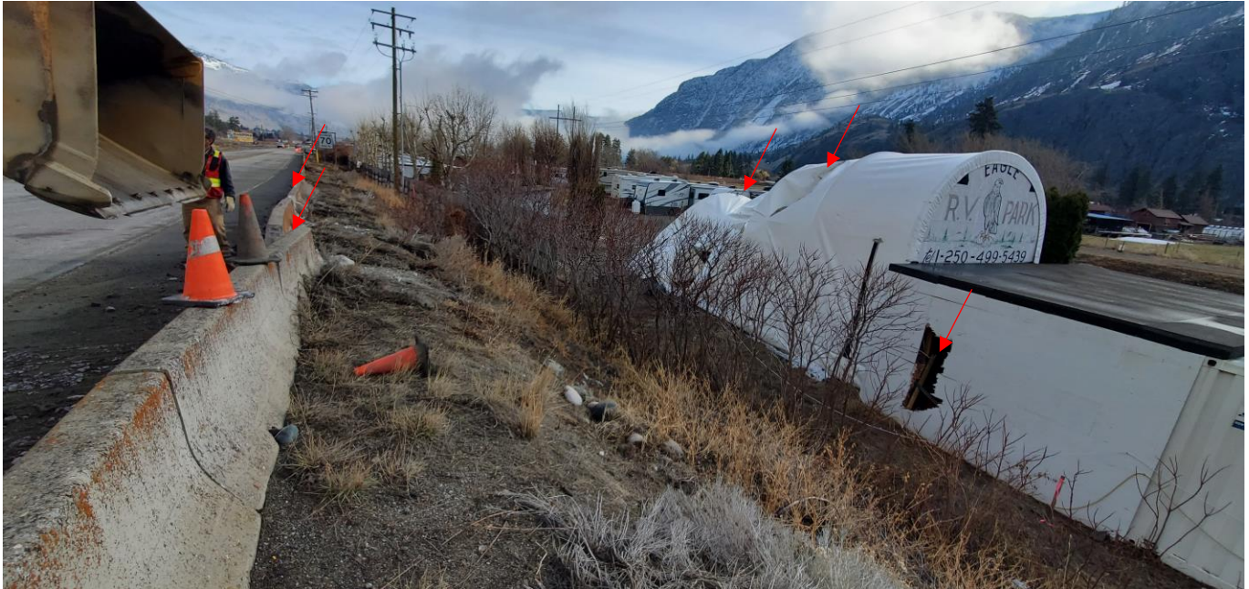
Photo 7 View of rock fall impact locations on concrete barrier and storage structures downslope.
