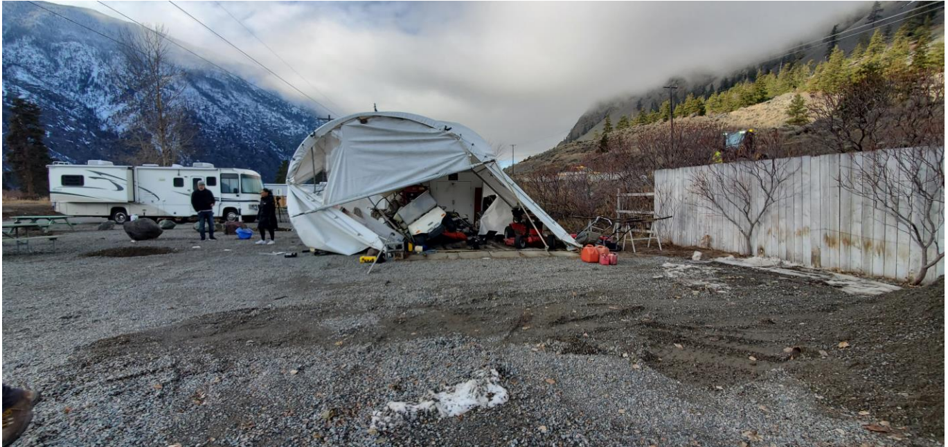
Photo 9 View of impacted storage structure, looking west.
