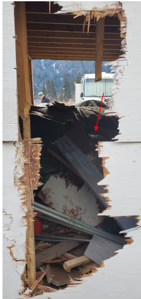
Photo 8 View of rock fall impact on wooden storage structure. Rock was located inside structure.
