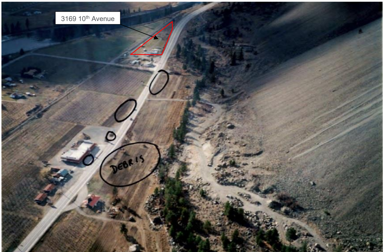
Photo 2.3a Photo of talus fan and rock fall debris locations from February 9 th , 1998 rock fall event looking west.
