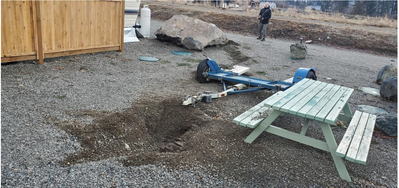
Photo 11 View of ground impact from Rock Fall #2, looking south.
