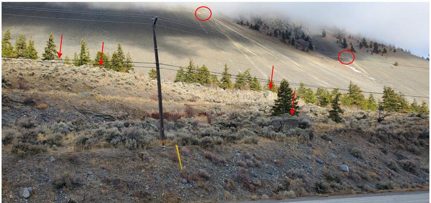
Photo 4 View of highway cut slope and talus fans above 3169 10 th Avenue. Rock fall greater than 1 m diameter indicated by red arrows. A portion of January 16 th rock fall boulders indicated by red circles.
