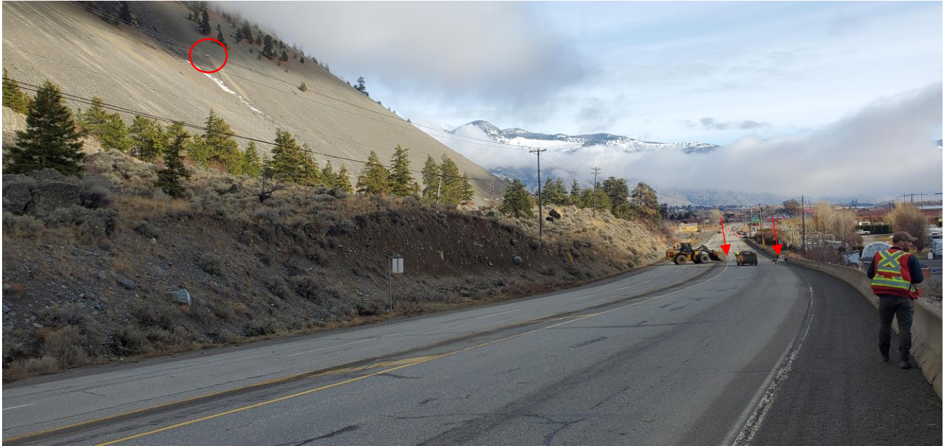
Photo 5 View of Highway 3 and associated soil cut slope above 3169 10 th Avenue. Rock fall impacts located at service equipment. Recent rock fall boulder indicated by red circle.
