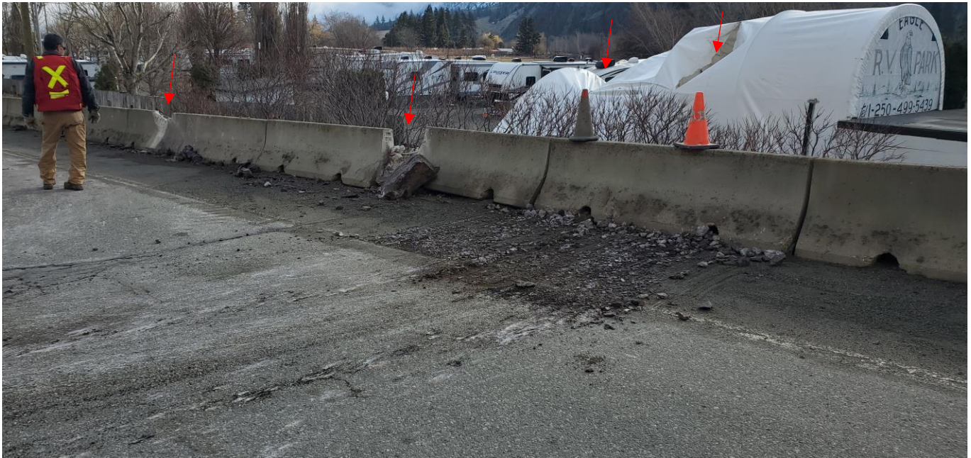
Photo 6 View of rock fall impact locations on concrete barrier and storage structure downslope.
