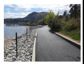
Erosion protection measures have been built into the project to reduce the impact of high water levels. Root barriers have also been installed next to trees to maximize the longevity of the asphalt path. This project was partially funded by the Province through Disaster Financial Assistance.
