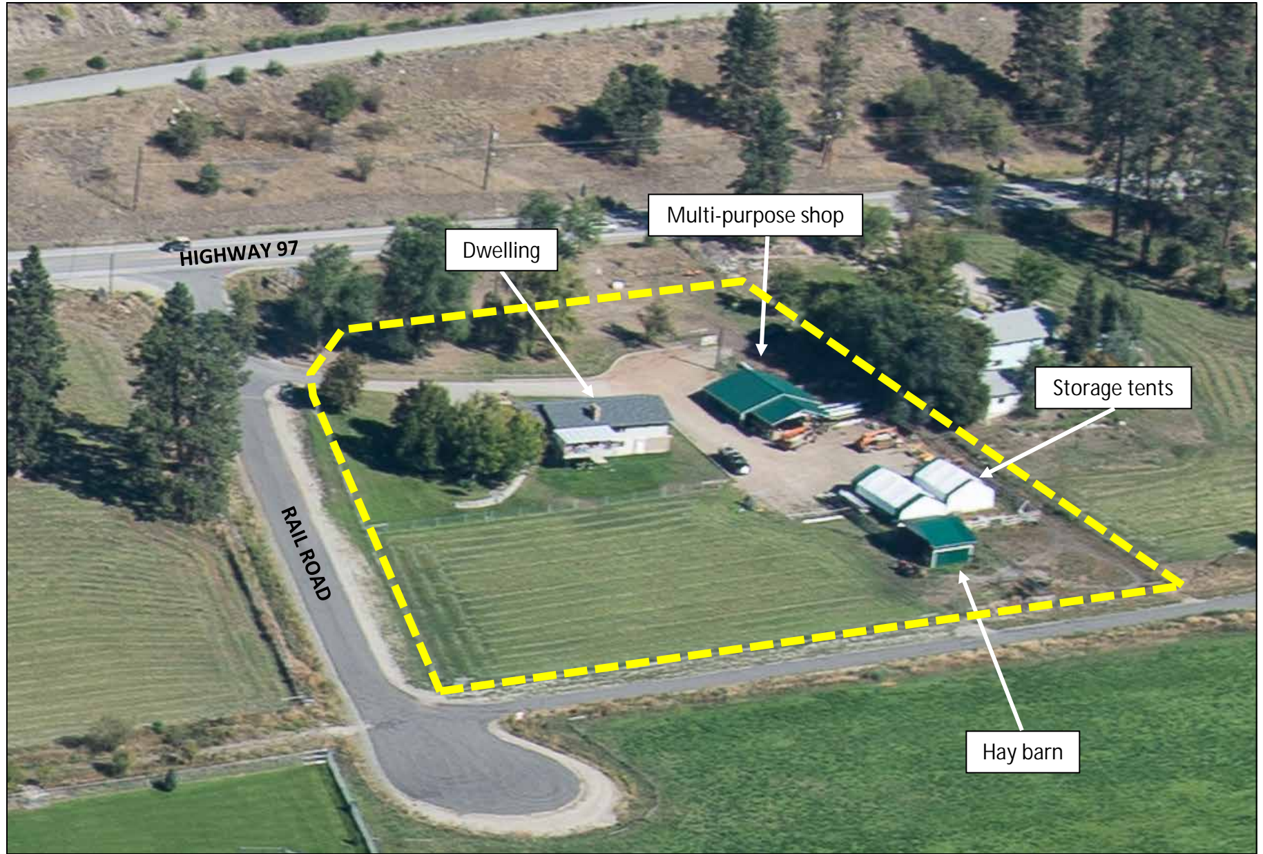
Attachment No. 1 – Aerial Photo (2014)
