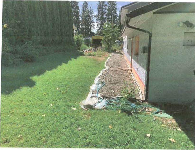
Photo 7 Looking south along east building wall at lot grading towards the structure
