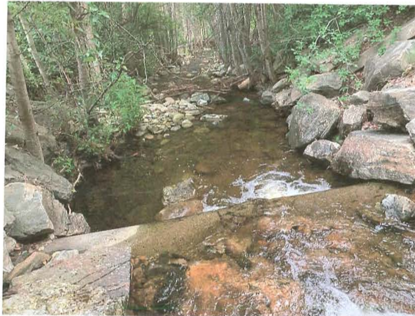
Photo 6 Looking downstream at weir below 8 th Street bridge and view downstream
