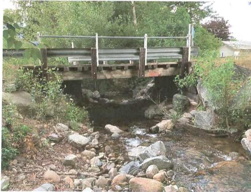
Photo 4 Looking downstream from left bank at 8 th Street bridge
