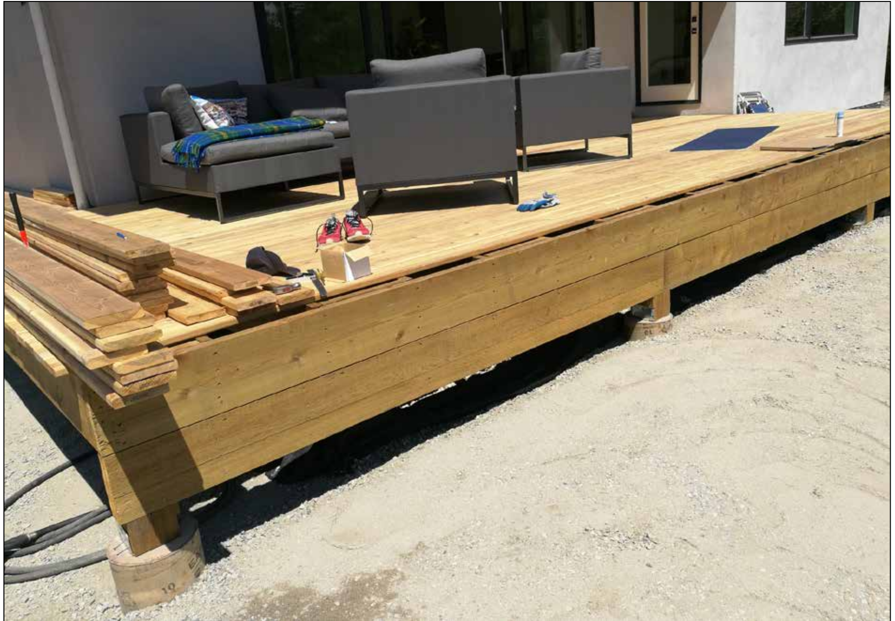
Attachment No. 1 – Deck Photo (2019)
