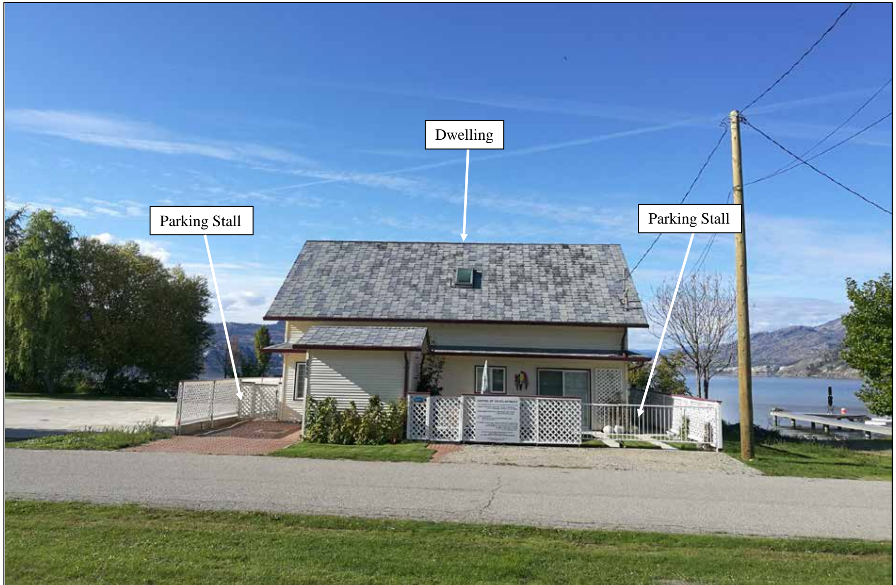
View of Subject Property from 1 st Street
