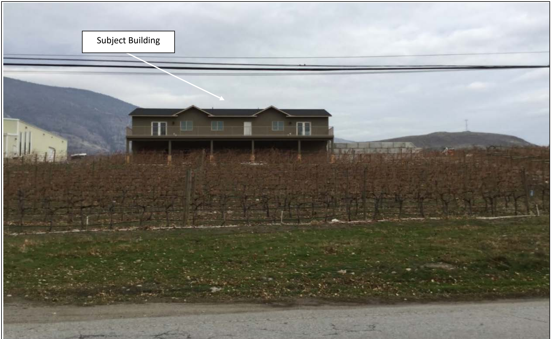
View of Subject Property Looking East from Tuc-el-nuit Drive
