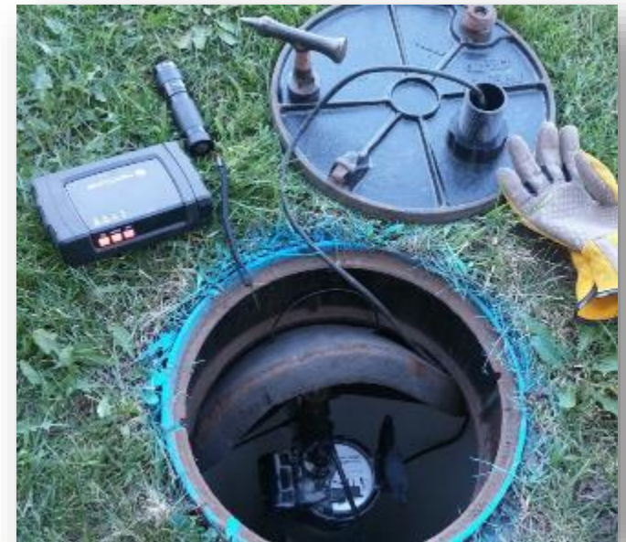
RDOS Award Winning Homeowner Leak Detection Program
